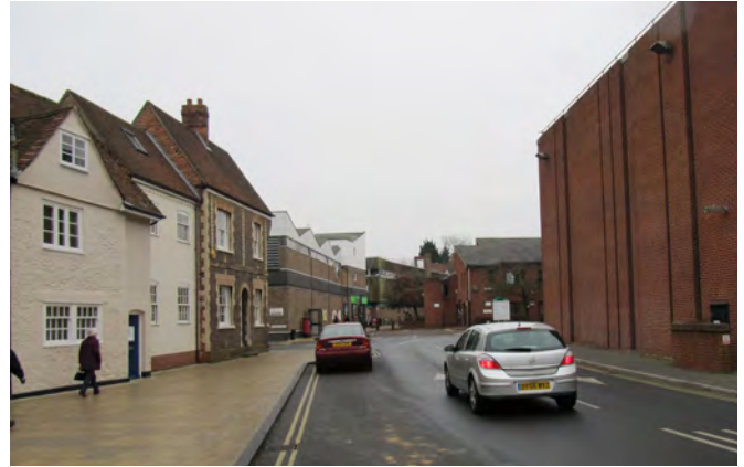
Fig 2.33: The group of buildings forming the former Bee Public House (left) opposite the multi storey car park (right)
