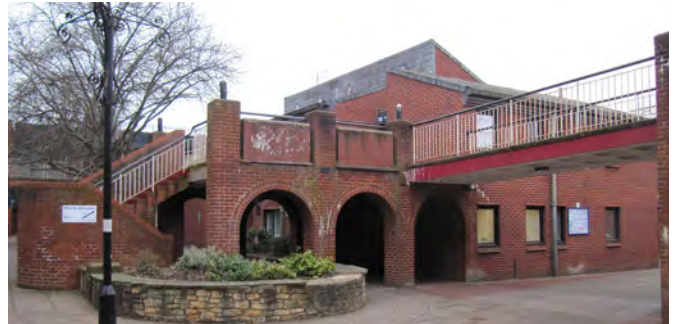
Fig 2.22 The Charter Area can be confusing and hard to navigate for pedestrians
