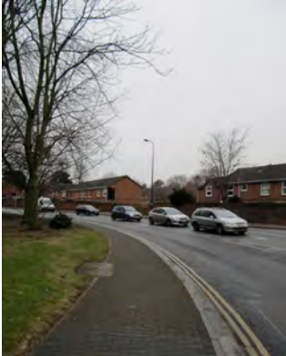
Fig 2.3 Stratton Way is a large, busy main road.
