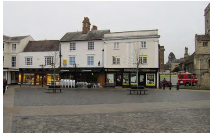
Fig 2.37: The group of listed buildings that front onto both the Market Place and Stert Street
