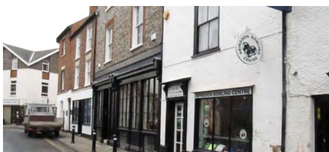
Fig 2.31: Brick and render might be used next to each other but rarely do they appear together on the same building.
