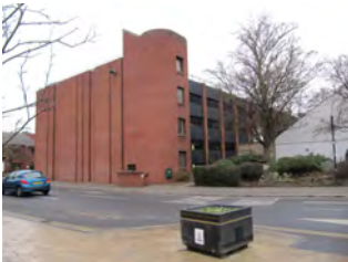
Fig 2.4 The Charter Area Car Park currently provides 474 parking spaces within the town centre
