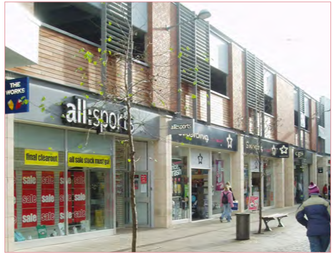
Fig 3.4: This development in Boston, Lincs creates a strong vertical rhythm that deflects attention from the parking on the upper levels
